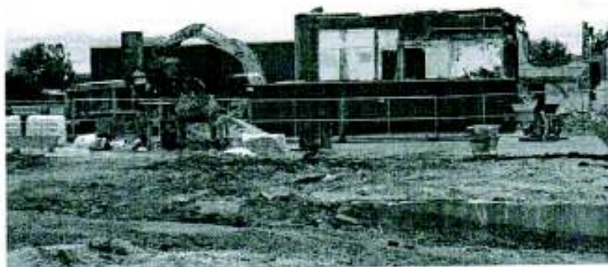
Demolition of the 1930's Onekama School for New Gymnasium and Cafetorium
