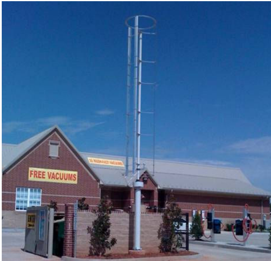
Windspire Wind Turbine Powering New Oklahoma City Eco Express Car Wash on 1825 East Memorial Road
