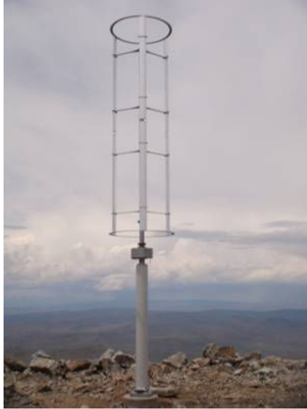
High Wind Windspire Installed atop a 9000' Mountain Peak in Nevada
