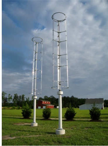
Windspire® Wind Turbines Installed in North Carolina
